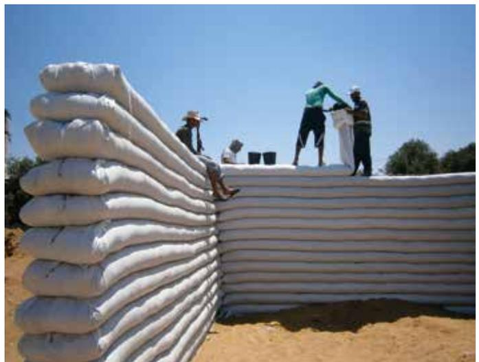
**Fig. 2** | Walls made with the Earthbag technique. Source: ARCò.
